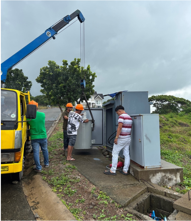
TRANSFORMER PLACEMENT
