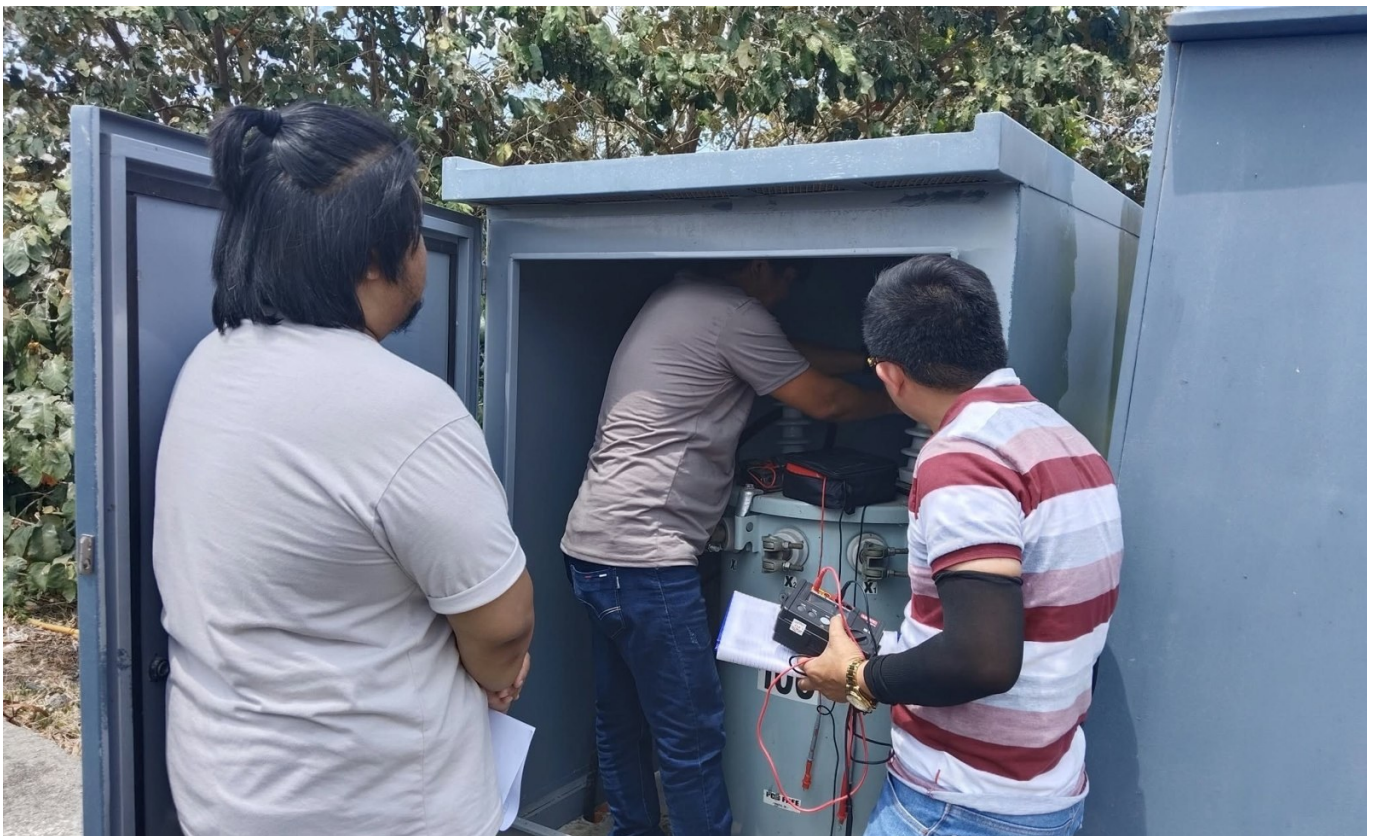
OCEAN HILLS SUBDIVISION / TRANSFORMER INSTALLATION
